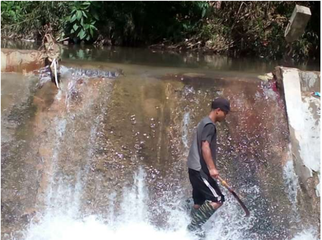
CLEANING WORK IN PROGRESS
