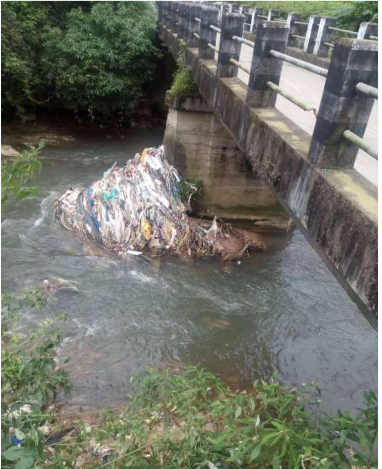
Fig4: Garbage carried by the river from upstream accumulated at the pillar of the bridge at Wahingdoh.
